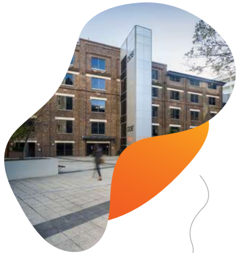
Ultimo Campus 46-52 Mountain St, Sydney
